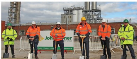
Pictured above (l-r): Mark Ellwood, Project Manager, John Turner Construction Group; Jeff McMeans, Project Engineering Manager, Ingevity; Norman Keane, Director of Innovation, Engineered Polymers, Ingevity; Steve Hulme, Vice President, Engineered Polymers, Ingevity; Graham Carr, Head of Warrington Laboratory, Ingevity; and Dwayne Taylor, Contracts Director, John Turner Construction Group.
